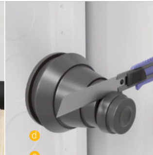
4. Installation of rubber gaskets
