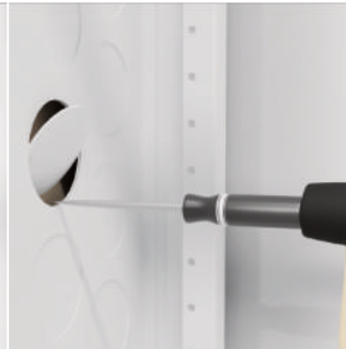
3. Blocking to pipes
