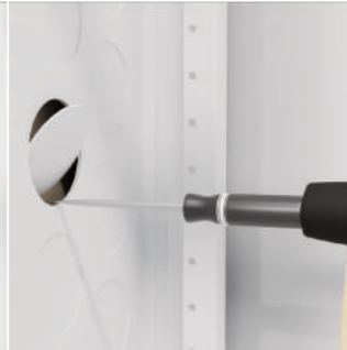
3. Blocking to pipes
