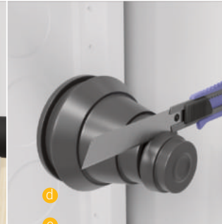
4. Installation of rubber gaskets
